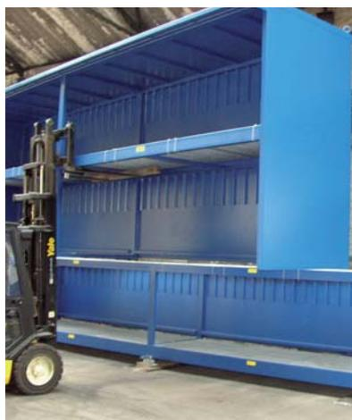
Installation of the 3P814 with ready-mounted container cover. Construction of the complete storage container is carried out in two parts.
